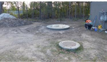
The top pictures show the old tank being dug out, and then out. The bottom pics show a big hole for the new tank covered by shadows, then the new tank installed.
