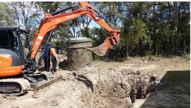
When the septic tanks were originally installed something obviously went amiss with accounting for future use. Our membership has now outgrown the designed use of the system installed and council has now decided that it may be cheaper to replace the existing system with a much larger tank rather than continually pumping it out. The works were done on 16 and 17<sup>th</sup> of September and the shed was totally closed over these two days.
